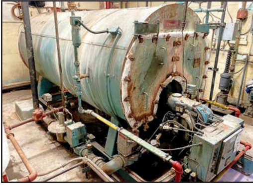
CLEAVER BROOKS CBE-200-60 STEAM BOILER
