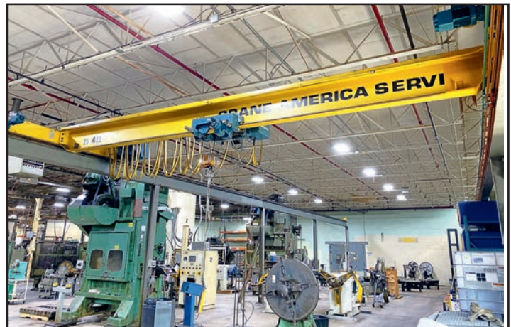
CRANE AMERICA SERVICE 5-TON FREE STANDING BRIDGE CRANE SYSTEM, APPROX 25' SPAN X 108' RUNWAY
